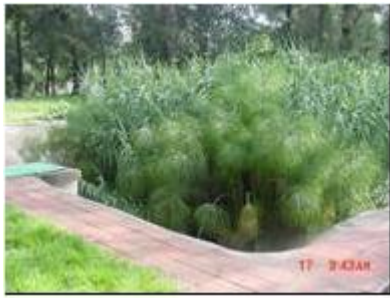
Figure 7a. UNAM Coyoacán Vivarium subsuperficial horizontal flow artificial wetland [23]
