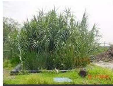
Figure 7b. UNAM Cultural Zone subsuperficial descending vertical flow artificial wetland [23]
